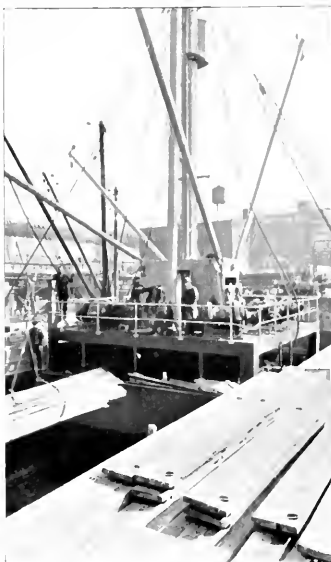
Westinghouse electric cargo winches handling Pacific Coast lumber at an Atlantic Coast terminal from the motorship Seekonk. Fuel cost 3 of a cent per ton handled.
